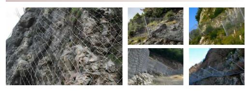
Slope protection net is a protective structure used to prevent natural disasters such as slope landslides and landslides. It is made of materials with excellent weather resistance and corrosion resistance, which can effectively fix soil and rocks, prevent soil erosion, and protect the stability of slopes. Slope protection nets are widely used in roads, railways, water conservancy, mining and other projects, playing an important protective role.
