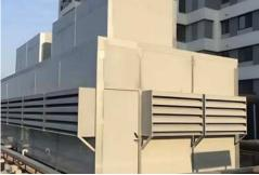
The equipment noise reduction barrier is a sound insulation structure specially designed to reduce the noise generated by the equipment. It is designed to effectively reduce the noise generated when the equipment is running and provide a quiet working environment. By using efficient sound insulation materials and scientific structural design, noise transmission is effectively reduced and the surrounding environment and personnel health are protected.
