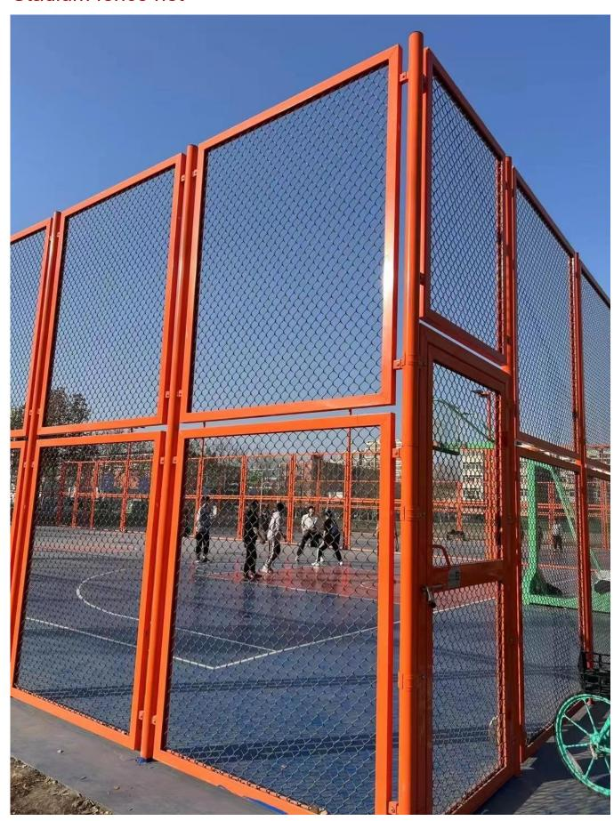
The height of the fence on both sides of the tennis court is 4-6 meters, with 4 meters at both ends. If the venue is adjacent to residential areas or roads, its height should be uniformly above 4 meters. In addition, a fence with a height of H=0.80 meters can be set up on the side of the tennis court to make it easy for the audience to watch the game. The height of the blocking net on the rooftop tennis court is over 6 meters.
